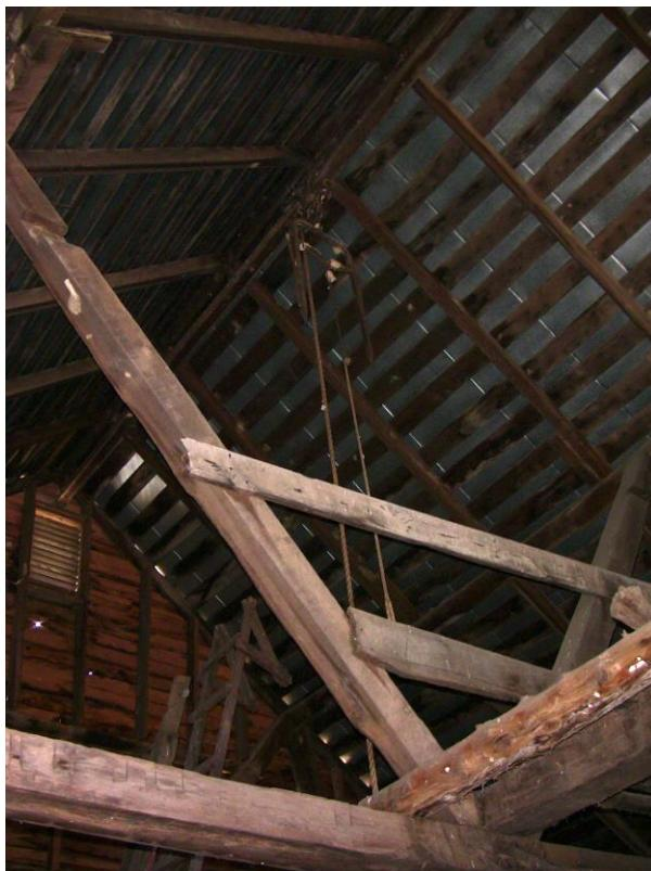
This is the apparatus described above. There is a track attached to the ridgepole, which extends outside the barn roof through the hay maw door. Note the carriage that moved along the underside of the track. Next note the rectangular two-pronged hayfork that was used to lift square hay bales. This was the last incarnation of the hayfork. It came along with the small square hay baler after World War II, and was replaced by the hay bale escalator.
