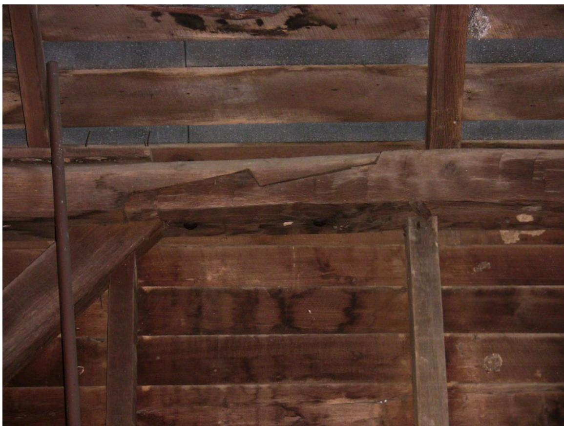
In the photo above, note the remarkably designed and masterfully executed joint that held two trusses of the top plate of the side wall framing, and which supported the horse barn's roof. Not seen, these two beams were held together by dowels. This joint was immune to stress applied from any angle. Its cultural origins are in Finland. One can watch one being made on a film produced by the Finnish Government's cultural division on YouTube.(6)
