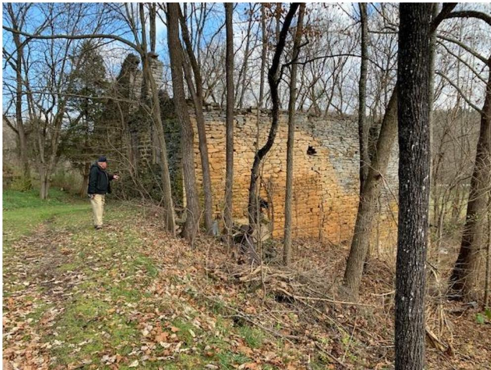
The author is standing on the filled in ditch that contains a two-foot diameter rolled and riveted iron culvert millrace that carried water from the creek above the mule barn to the flourmill. This pipe entered the stone masonry of the second floor and fed the water wheel which was entirely enclosed within the lower floor. Note the lighter colored stone in the building's wall, indicating that it had once fallen in, and was rebuilt.
