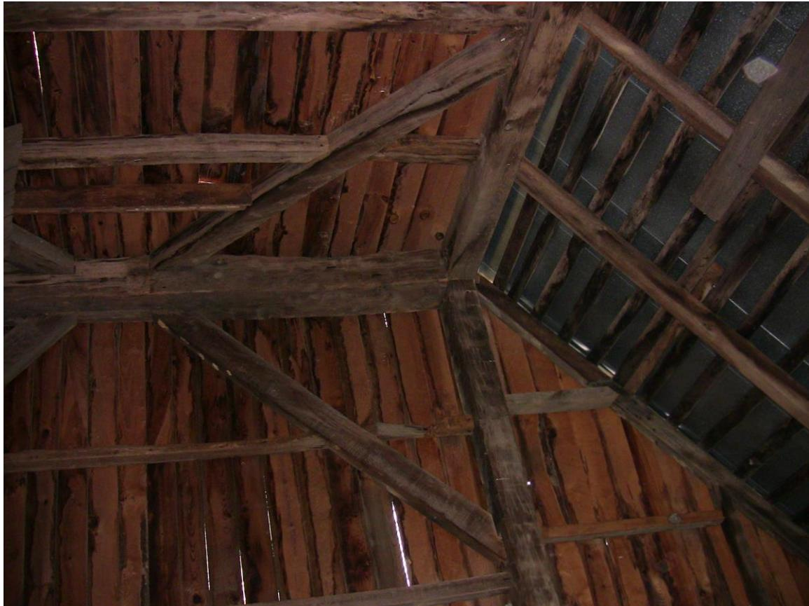
In the two photographs below continue to note the carved joints that fasten the smaller beams into the larger ones, and the dowels that are driven into gimlet (old name for a hand auger) bored holes. From the angle of the hewing marks on the larger beams one can tell that the worker was right handed. The degree to which the carpenter understood the distribution of stress supported by these angled beams is truly admirable.
