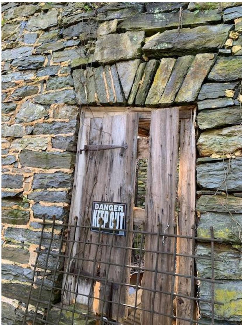
Note that some of the stone joints are held in place by quick lime mortar, and some are necked.
