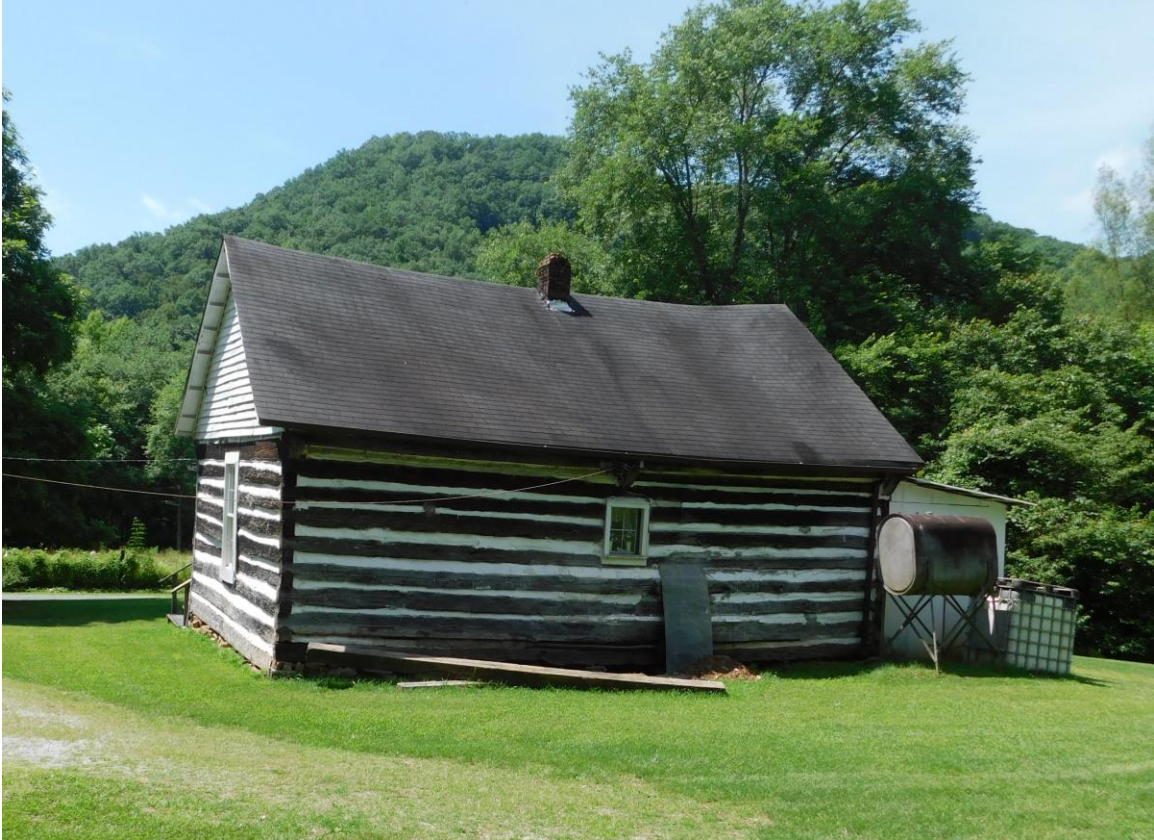
THE REAR OF THE CHURCH NOTE THE SAG IN THE PEAK OF THE ROOF AND THE CENTRAL INTERNAL CHIMNEY
