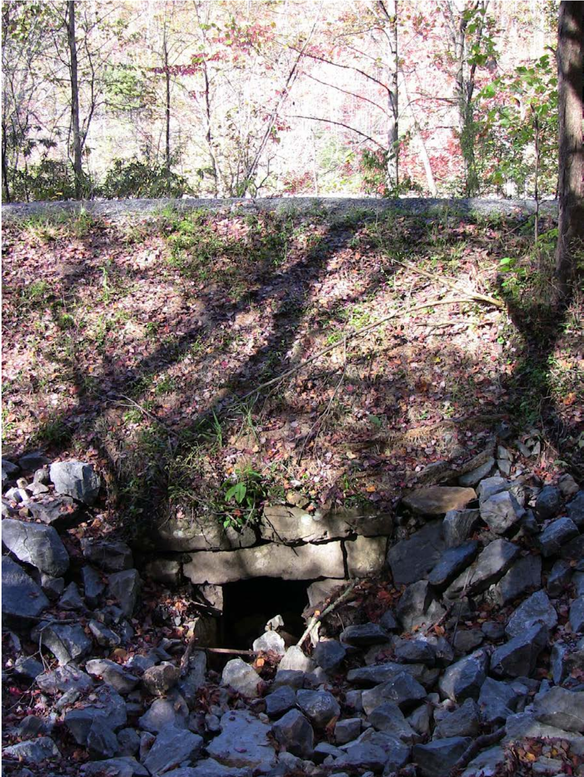
The original culvert under the L&N RR track, made from cut stone
